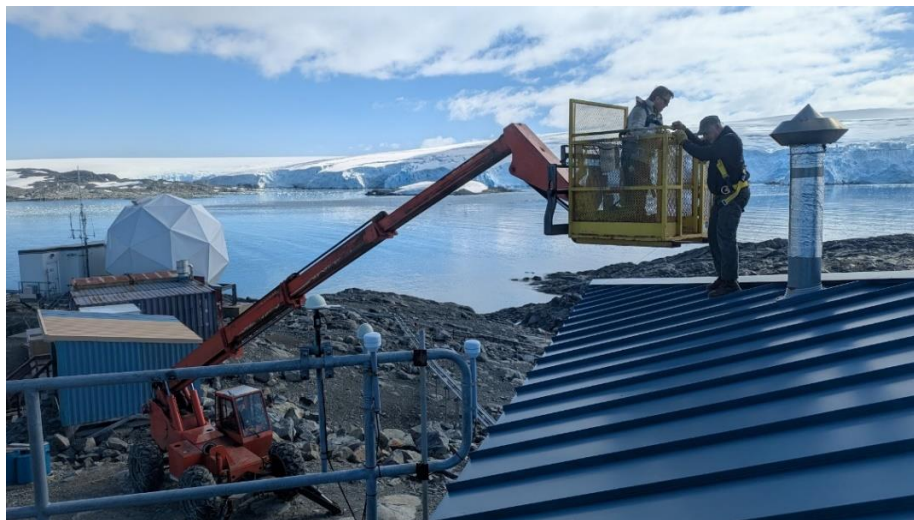
Figure 20. Carpenter and Maintenance Specialist replacing the RASA inlet on the Terra Lab roof.
